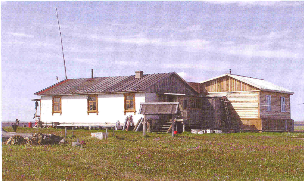
Fig. 4: Samoylov Station on Samoylov Island (Lena Delta) showing the main building on the left and the new extension on the right side (G. Stooß, AWI).
