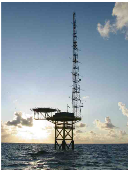
► Figure 5 Research platform FINO-I with its ~101 m tall measurement mast. The marine radar is located below the helicopter deck. The radar-image sequences depict a wave field propagating in easterly direction.
