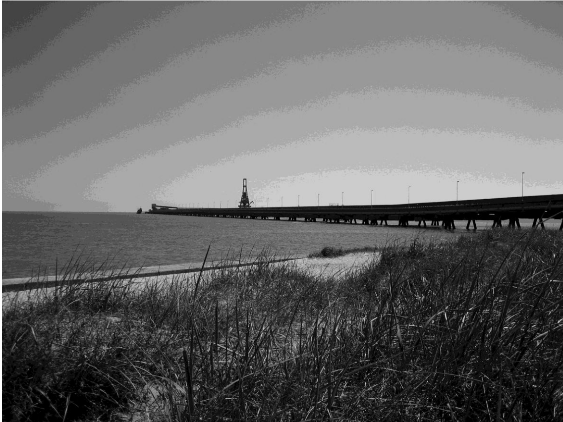
Fig. 2: Cargo bridge Niedersachsenbrücke in the Jade (JD) estuary where mussels were cultivated nearshore on suspended substrates using harnesses hanging from the bridge (2007).
