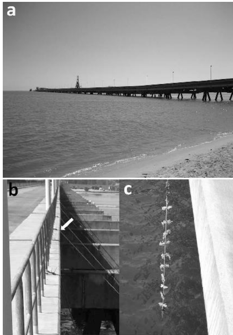
Fig. 2a-c: (a) The 1,300 m long cargo bridge at the Jade estuary, (b) harnesses attached to a steel beam, hanging between the pillars of the bridge (see white arrow), each of them consisting of (c) a 20 mm rope carrying substrate samples and a weight at the distal end.
