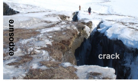
Fig. 1.8: Photograph of the crack. Picture by D. Fortier.
