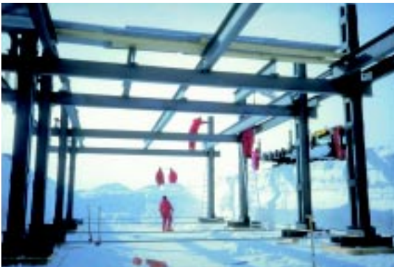
Fig. 4: Construction of the platform.
