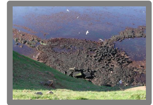
Beton, Basalt, Geröll
