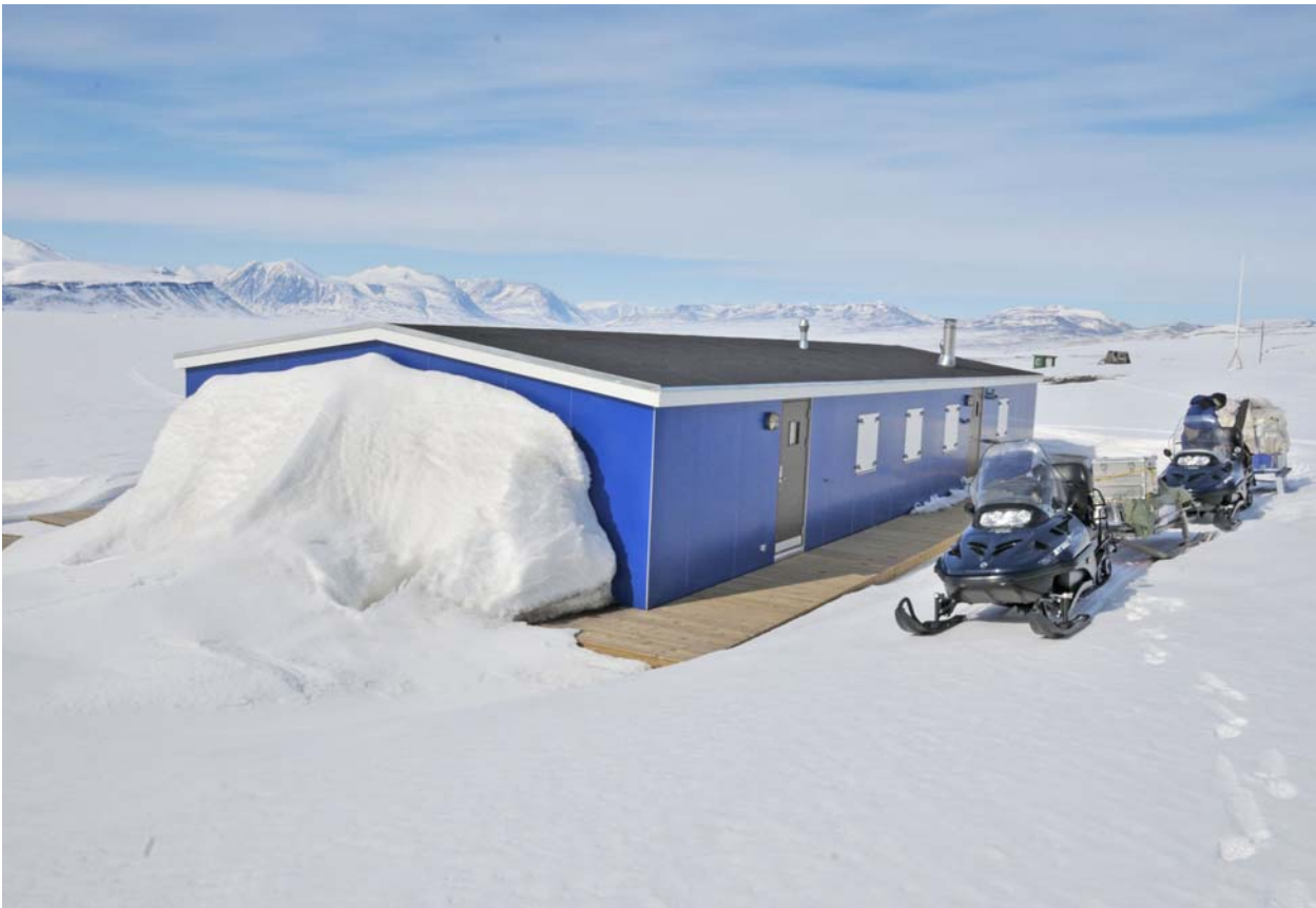
The new researcher house at Daneborg. Photo: Jøgen Skaftø.
