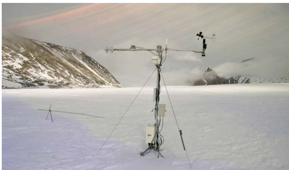
Figure 3.2 The AWS1 station as found in May 2010. The failed frame supporting the sonic ranger can be seen on the left. To counteract glacier flow, the station was entirely dug free from the snow cover and moved back to its original position of 2008. Photo: Michele Citterio, GEUS.
