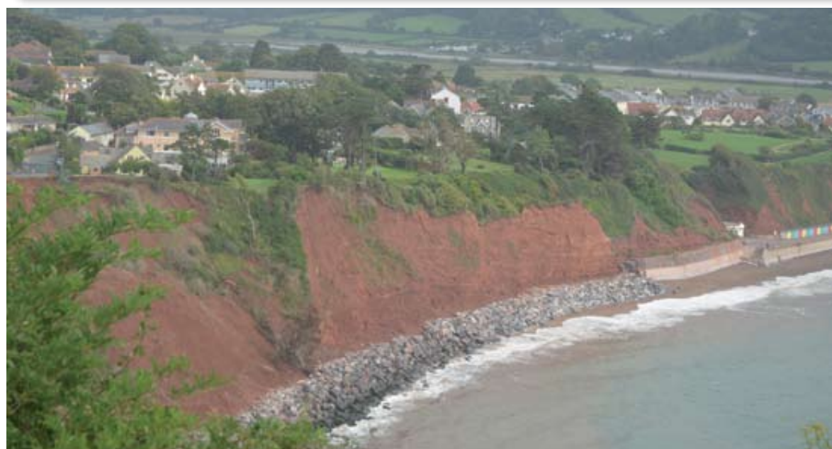
Triassic rocks exposed in the cliffs at Seaton looking east toward Axmouth and the River Ax. Blocks of limestone at the base of the cliff are to prevent erosion.
