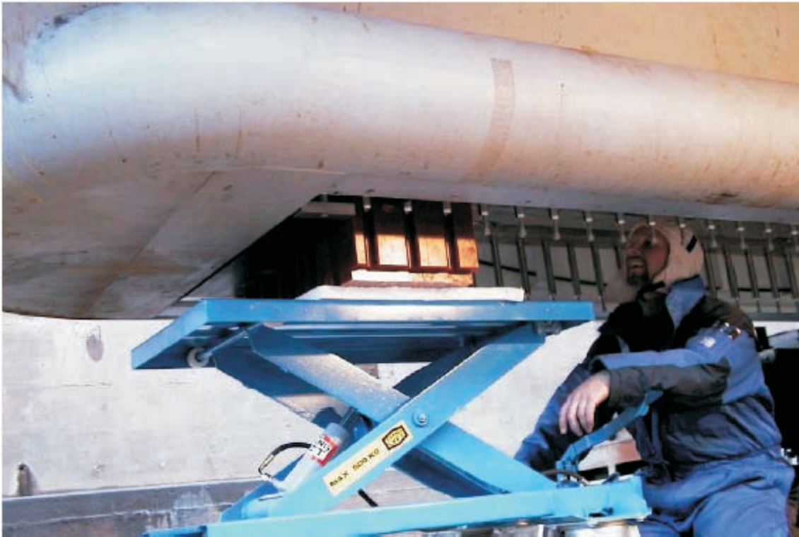
Figure 37 Flush installation blister for the EM 122
