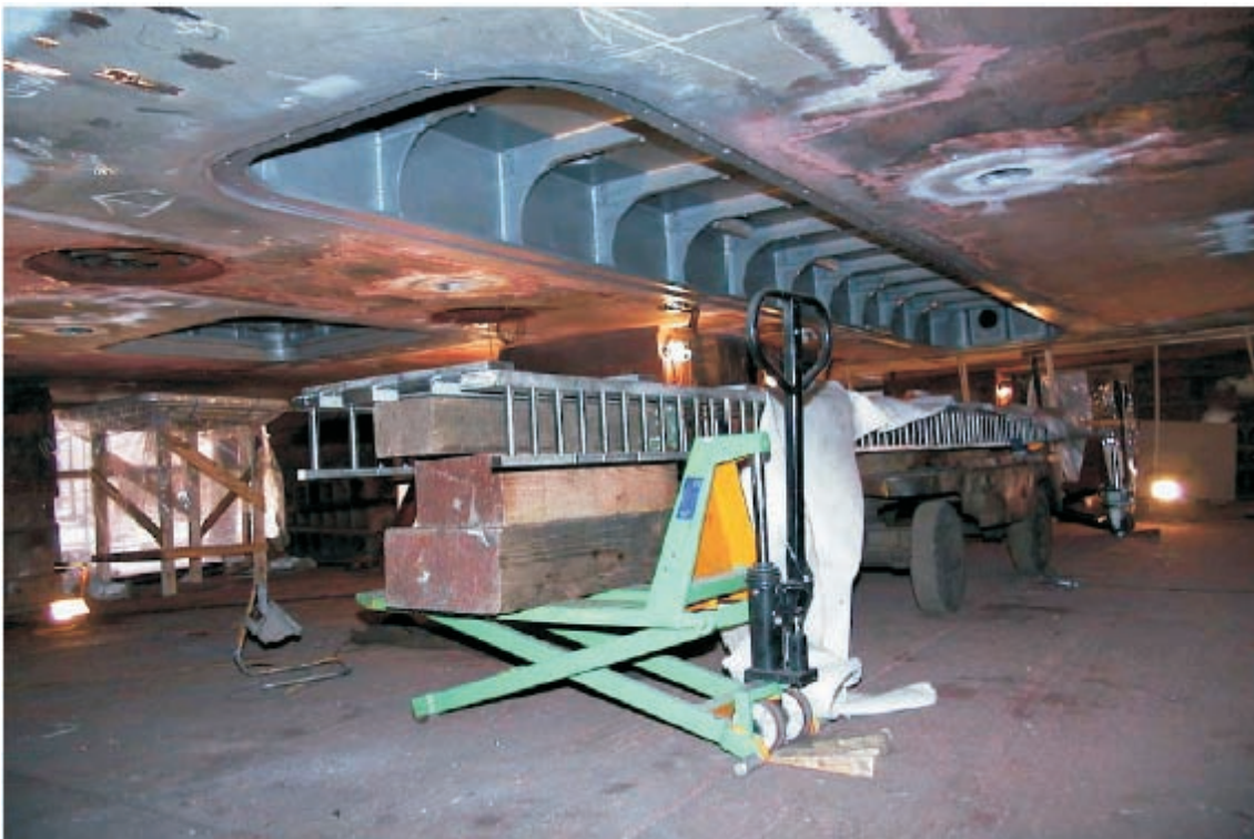
Figure 37 Flush installation blister for the EM 122
