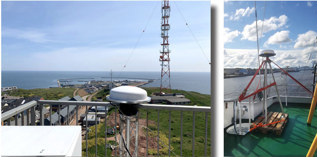
Fig. 2.3: Installation of the communication antenna on the Lighthouse Heligoland and on the Uthörn . By M. Brand and I. Bussmann
