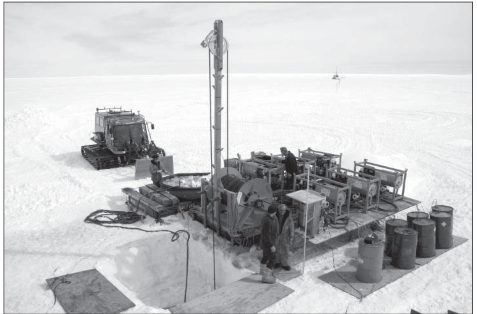
Fig. 2. Hot-water drill rig setup for hydrophone deployment. Pictured left rear to right front are a snowcat, the black meltwater basin with snow, a pressure hose and drill winch, six hot-water pressure washers on the drill platform, and fuel supplies in barrels. The actual borehole is at the bottom of the snow hole in the front. Penetrating the 100-meter-thick ice shelf with 700 kilowatts heating power took about 12 hours for each of the four holes. PALAOA's central instrumentation container is visible in the distant background.
