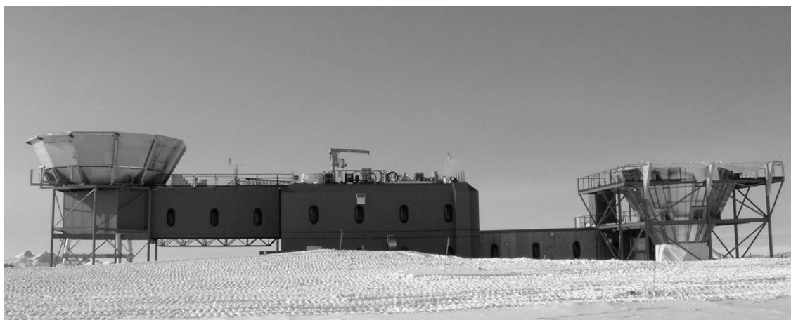
Figure 13-4: The MAPO Building. SPIREX and later DASI to the left, to the right is the Viper telescope, a 2.1-m off-axis telescope which hosted the ACBAR and SPARO instruments, used for CMBR studies and for mapping polarization at sub millimetre wavelengths, respectively. Image provided by the Office of Polar Programs, National Science Foundation.
