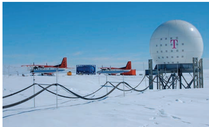
Fig. 11: Ground service and refuelling facilities at NM-II for smaller aircraft such as Dornier 228, Twin Otter and Basler BT-67. The radom (right) housing the satellite dish-antenna for the permanent satellite communication link (128 kbit s -1 ) is installed on a special support structure, which has to be extended regularly to compensate snow accumulation.
