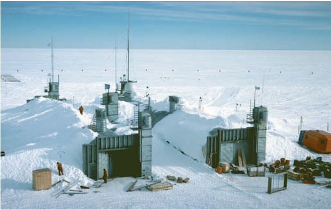
Fig. 3: Georg von Neumayer (GvN) research station built on the moving Ekström Ice Shelf at initial position 70^{\circ}37'S , 08^{\circ}22'W and commissioned on 3 March 1981. The photo shows the station just after completion of construction works. The concept is an underground station made of two parallel steel tubes, which accommodate containerised modules for a wintering team of four scientists, four technicians and one physician. The increasing loads of accumulating snow led to unavoidable destructions. The station lasted for eleven years and was replaced by the present Neumayer Station II (NM-II) during austral summer season 1991/1992.
