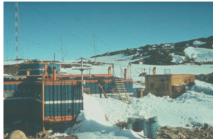
Fig. 2: Georg Forster Station in the Schirmacher Oasis at 70^{\circ}46'S , 011^{\circ}41'E , originally established as an annex to the Soviet station Novolazarevskaya, which was commissioned on 20 April 1976. At that time the construction concept was pioneering. Prefabricated container modules for laboratories, small power plant and accommodation were carried on sledges from the unloading site at the ice edge of the Lazarev Ice Shelf over a distance of 120 km into the Oasis. There the base was assembled on rocks within six weeks. Figure shows the base after the first wintering. In forefront the main building consists of six modules. The power plant on the right side is separated from the compound because of safety reasons. One module close to the antenna mast accommodated the radio transmitting system for ionospheric studies. The station was used until 1993 and then dismantled in the frame of a German-Russian project, which was completed in 1996.
