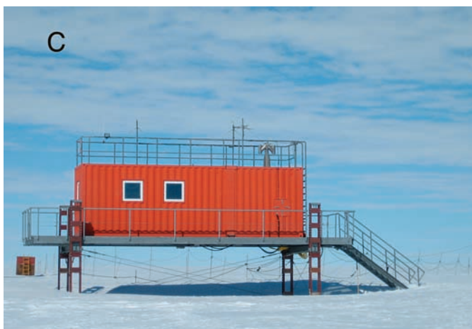
Fig. 6: Outside observatory structures at Neumayer Station II (NM-II) for meteorological, air chemical and geophysical investigations, measurements and data recording.
