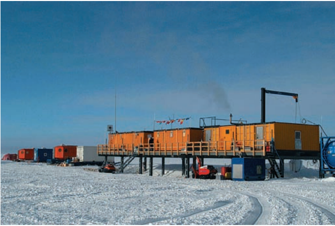
Fig. 9: Kohnen Station is the southernmost outside facility, which has to be supplied via NM-II. Small aircraft such as Basler BT-67 provide access to the station early in the season in order to extend the operational period. The main building of Kohnen Station consists of a 32 x 8 m platform on steel pillars on which eleven prefabricated container modules are mounted. Up to 25 persons can be accommodated.
