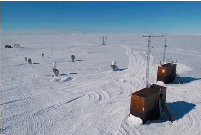
Fig. 4: The present Neumayer Station II (NM-II) on the Ekström Ice Shelf (initial position 70^{\circ}39'S , 008^{\circ}15'W ) was commissioned in 1992. The station is meanwhile covered by c. 9 m of accumulated snow, and will bear the increasing loads until 2009 at the longest. The photo shows the two stairway entries (foreground right), antennas and air ducts, the ramp to the garage section (left upper corner) as well as the wind power plant (background), which have to be extended periodically according to snow accumulation to keep access to the tubes below the snow surface. Presently the stairway towers have 96 steps.
