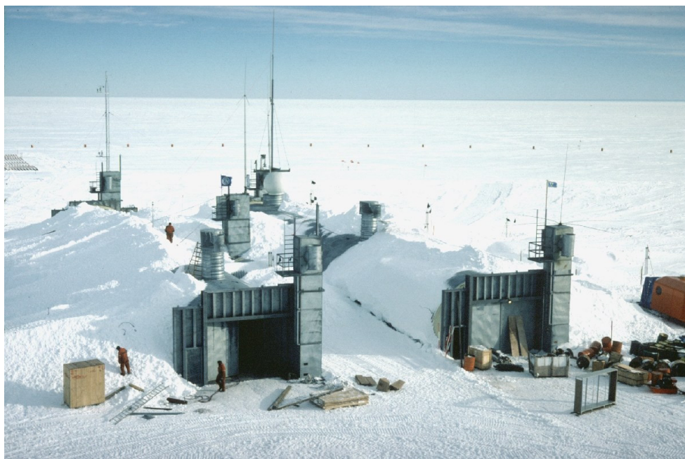
Fig. 5. The first Georg von Neumayer-Station , built underground on Ekström Ice Shelf near Atka-Bucht in 1981 for an overwintering team of 9 scientists and technicians. Archive AWI
