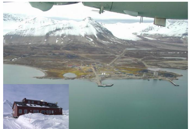
Figure 2-7: The high-latitude research station in Ny Alesund, Spitsbergen, photographed from the air. In the small picture on the left, the observatory containing our microwave radiometers is shown, which can also be made out in the middle of the larger picture. Pictures by M. Palm (IUP Bremen).
