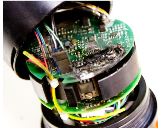
Figure 7: The damage of the MCT, likely caused by a leak in the tube.
