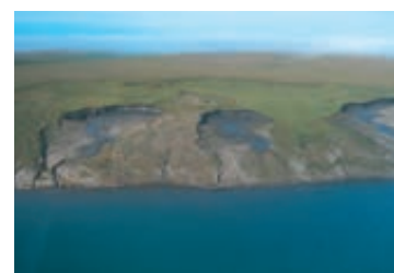
Along the Arctic Ocean fringe permafrost coasts are eroding, in some regions are losing up to 30 metres of coastline a year. Photos: H. Lantuit
