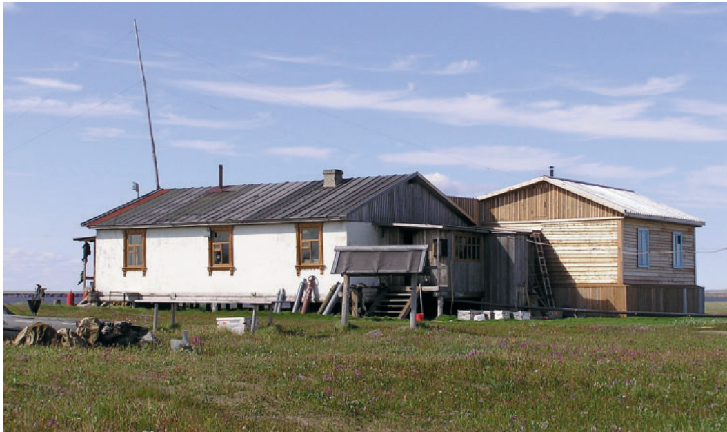
Fig. 4: Samoylov Station on Samoylov Island (Lena Delta) showing the main building on the left and the new extension on the right side (G. Stoof, AWI).
