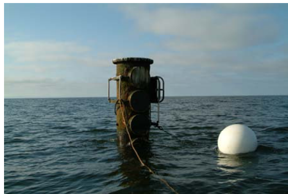
Figure 6: Single pile of the research platform ODAS, which serves as one longline connection.
